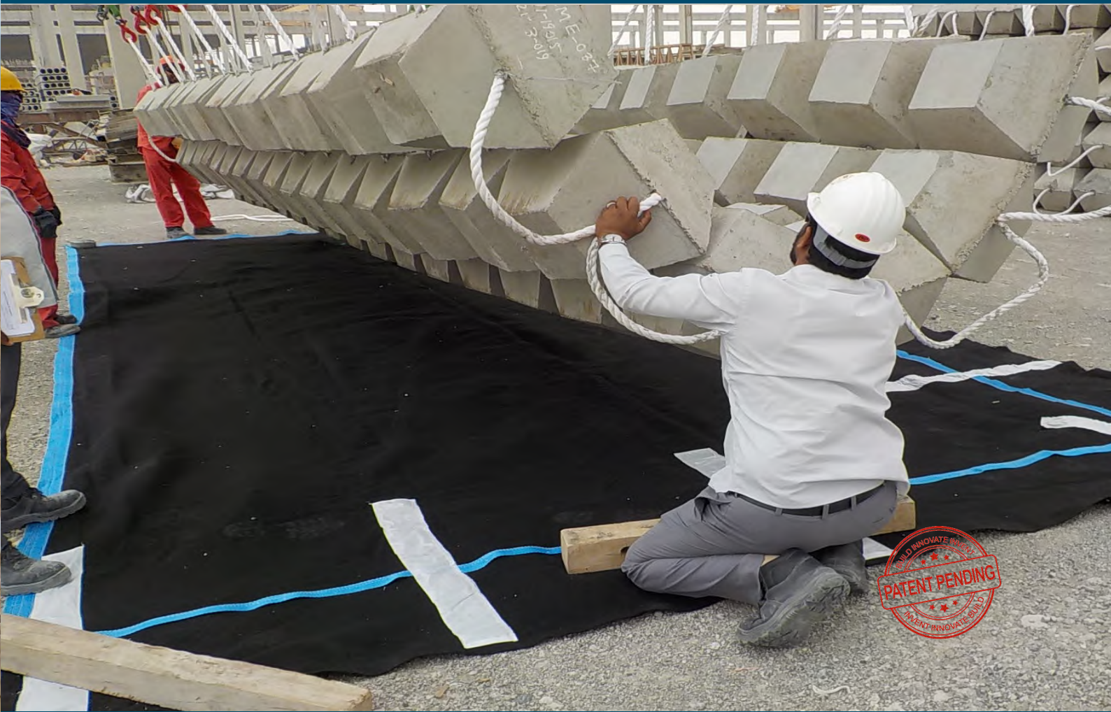
Concrete mattresses pre-fitted with GEO-MAT geotextile mattress
