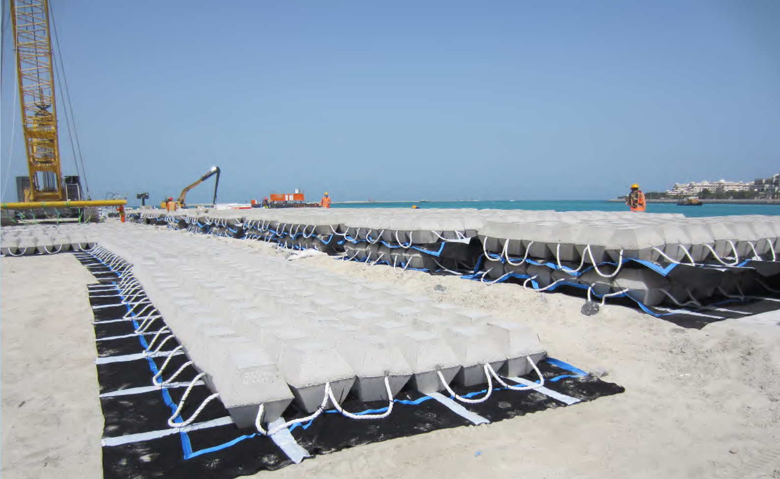
Concrete mattresses manufactured in situ prior to installation
