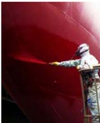
Epoxy based coatings dominate steel protection for marine exposed infrastructure
