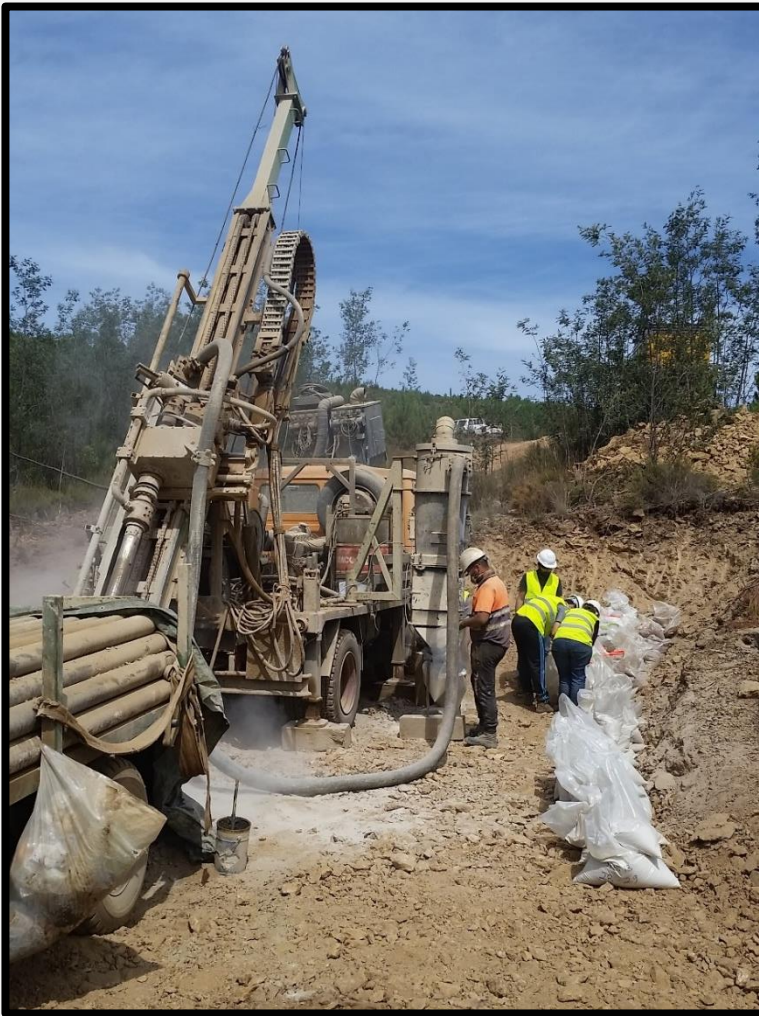
Figure 2. RC drilling at Reservorio
