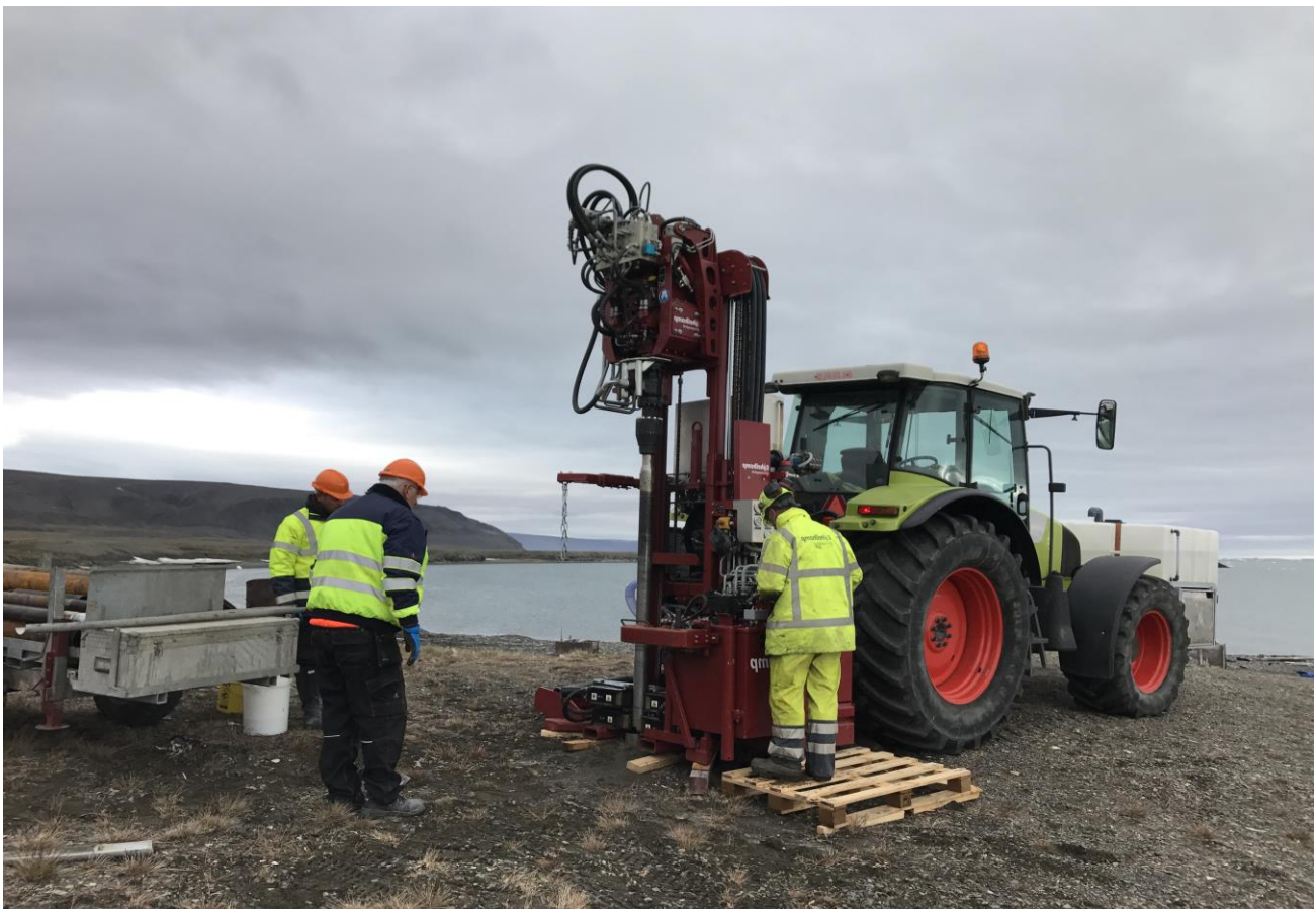
Figure 1. Sonic drill rig in operation
